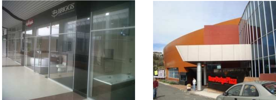
Figura 2.8 Almacén Bath Center Home Desing Plaza
