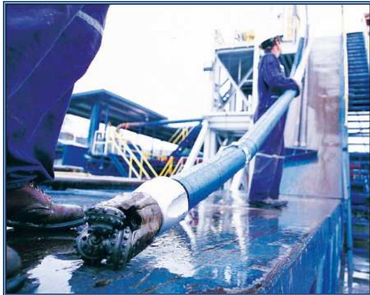
Figura.12 Herramientas del Pozo Horizontal Re-entry.
