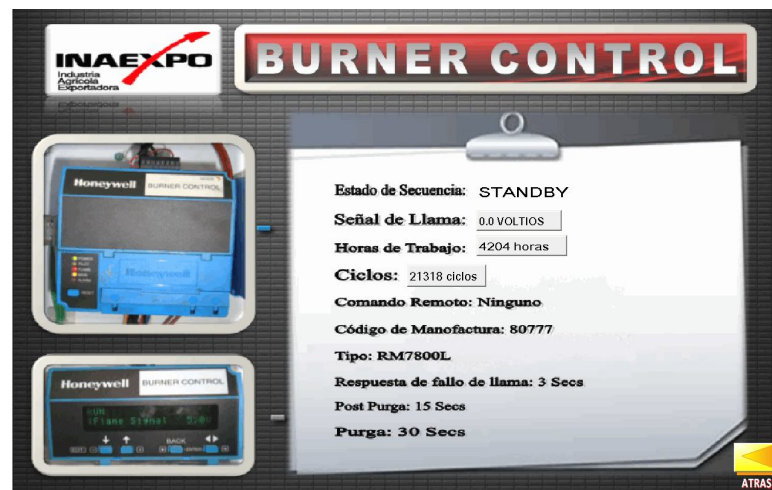
Figura 4.41 Pantalla Burner Control
