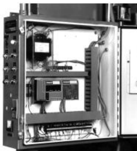
Fig. 7. Electrical panel installation.
