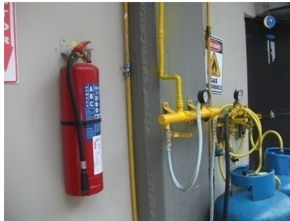
Figura 4.2: Centralina Gas
